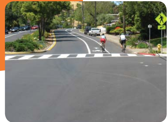
By narrowing the median, bike lanes were added providing a separate lane for cyclists without removing parking ( below ).
