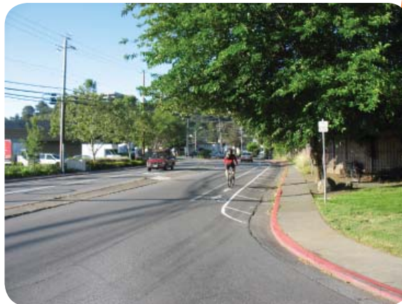
Adding bike lanes ( below ) provides a dedicated lane for cyclists on this busy street.
