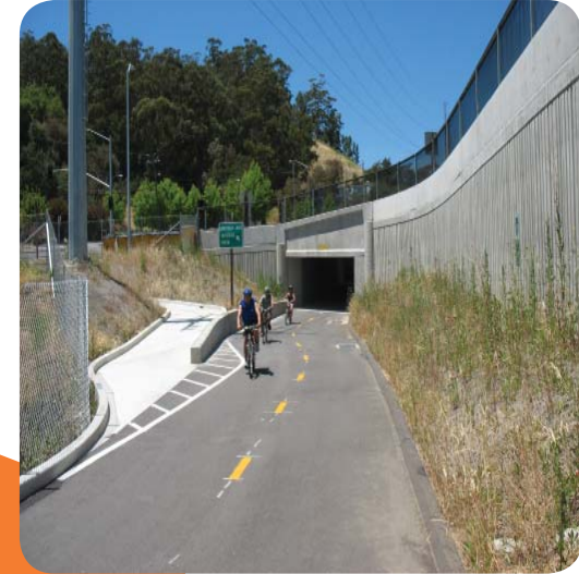
The tunnel under the Lincoln Avenue freeway ramps provides a safe separation from high-speed traffic for cyclists and pedestrians.
