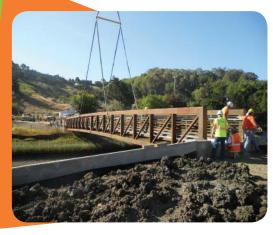
The centerpiece of an improved trail through the Tennessee Valley in Mill Valley, near the Dipsea Cafe, was slipped into place June 8, 2012. A concrete floor still needs to be poured on the 100-foot span, which opened June 15, 2012. The bridge was lowered into place by a hydraulic crane across Coyote Creek in Mill Valley.
