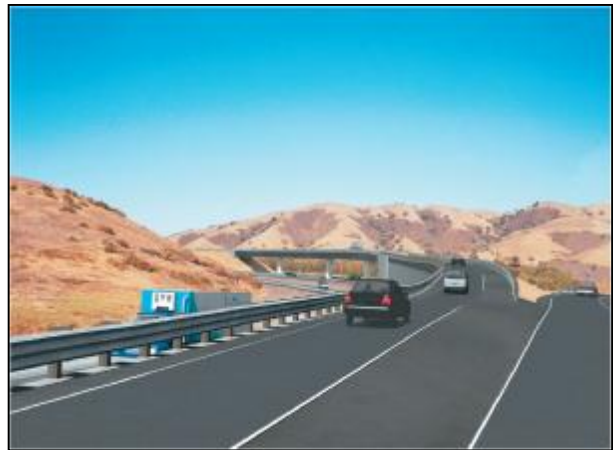
Figure 8: SR 152/156 proposed - grade-separated overpass facility
