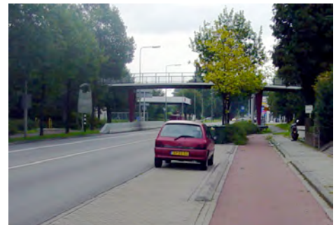
Figure 4: Bike path next to a parking lane
